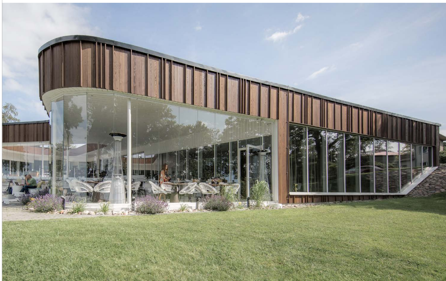
Oiled Thermory Benchmark thermo-ash cladding. NOA Restaurant in Estonia Photography Elvo Jakobson
