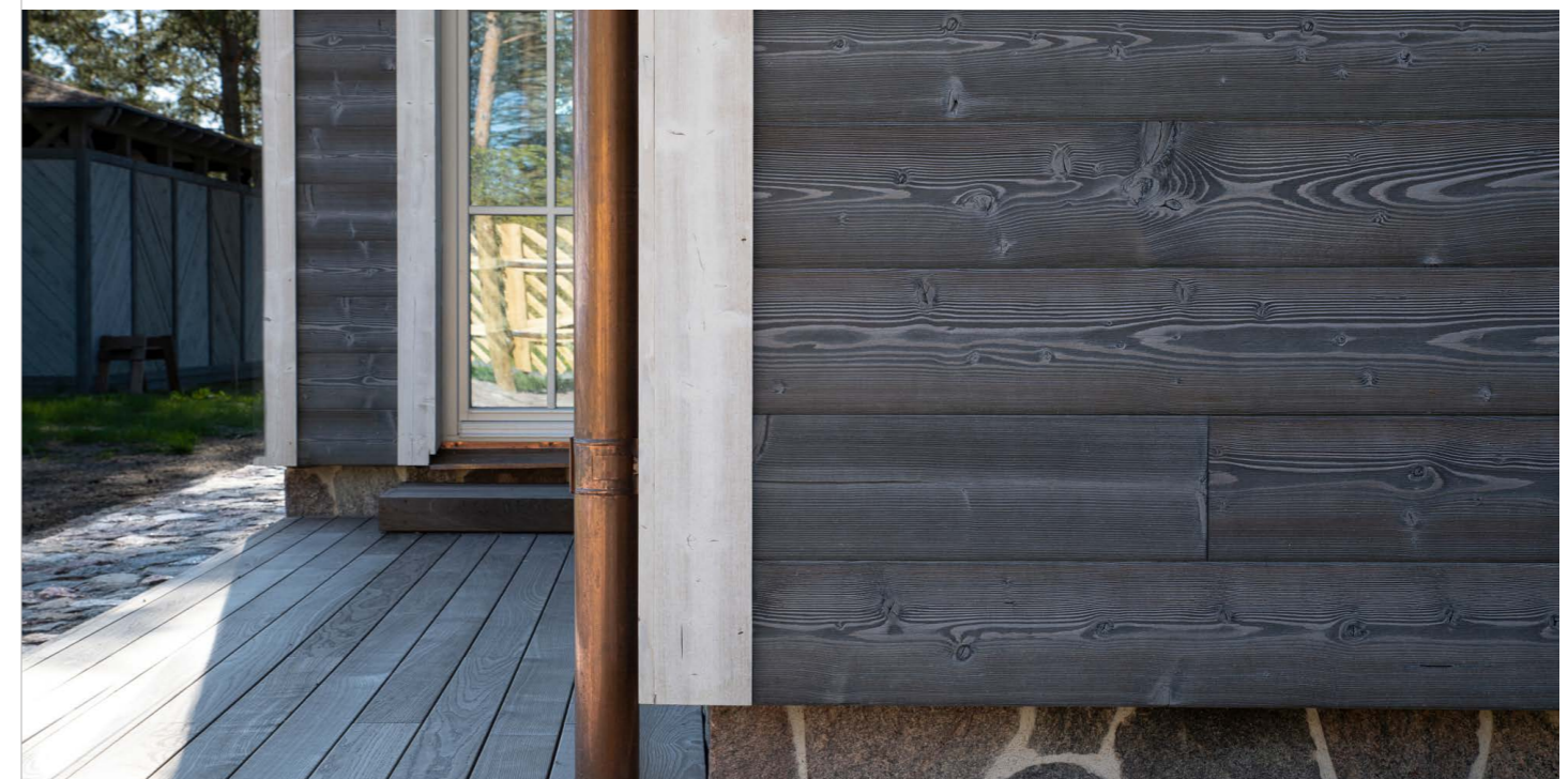
Drift Platinum and Sandy Pearl thermo-spruce cladding. Private house in Estonia Foto Aivo Kallas
